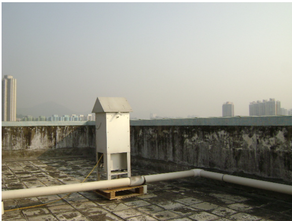
Roof top of Block 15, Yuet Wu Villa
