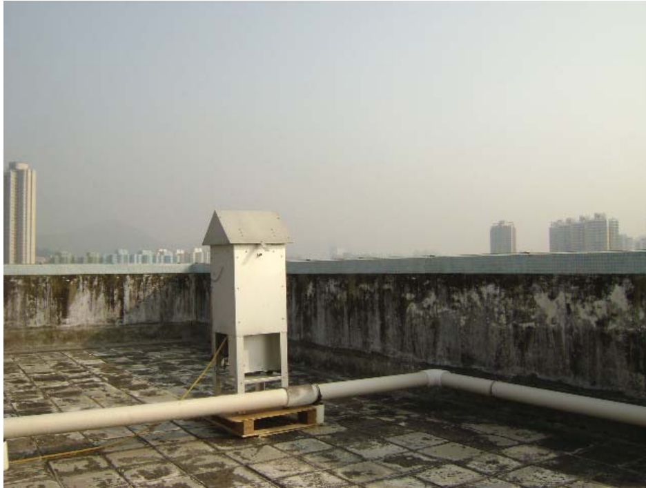
Roof top of Block 15, Yuet Wu Villa
