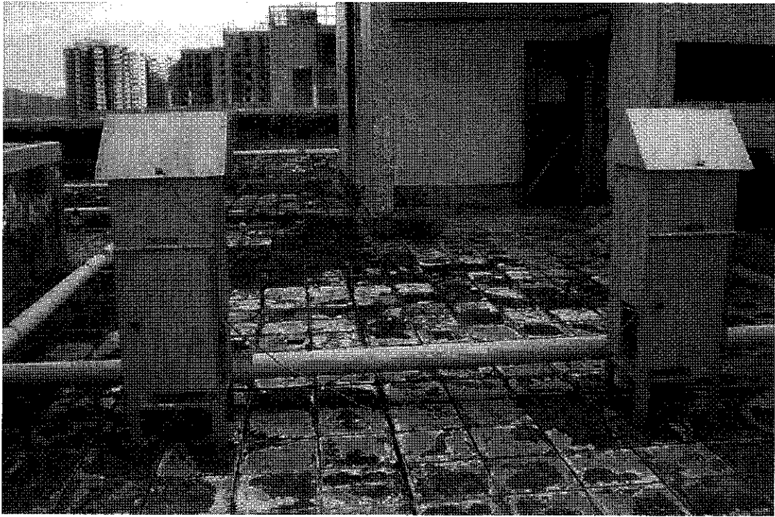
Roof top of Block 15, Yuet Wu Villa
